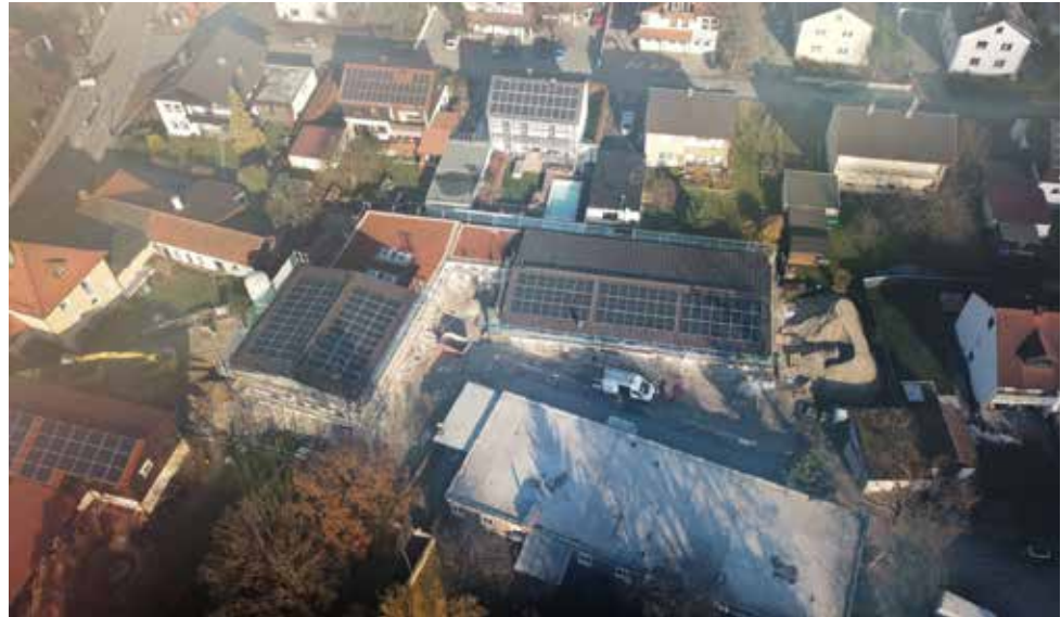
▲ Dachanlage Kindergarten Emmerting.
